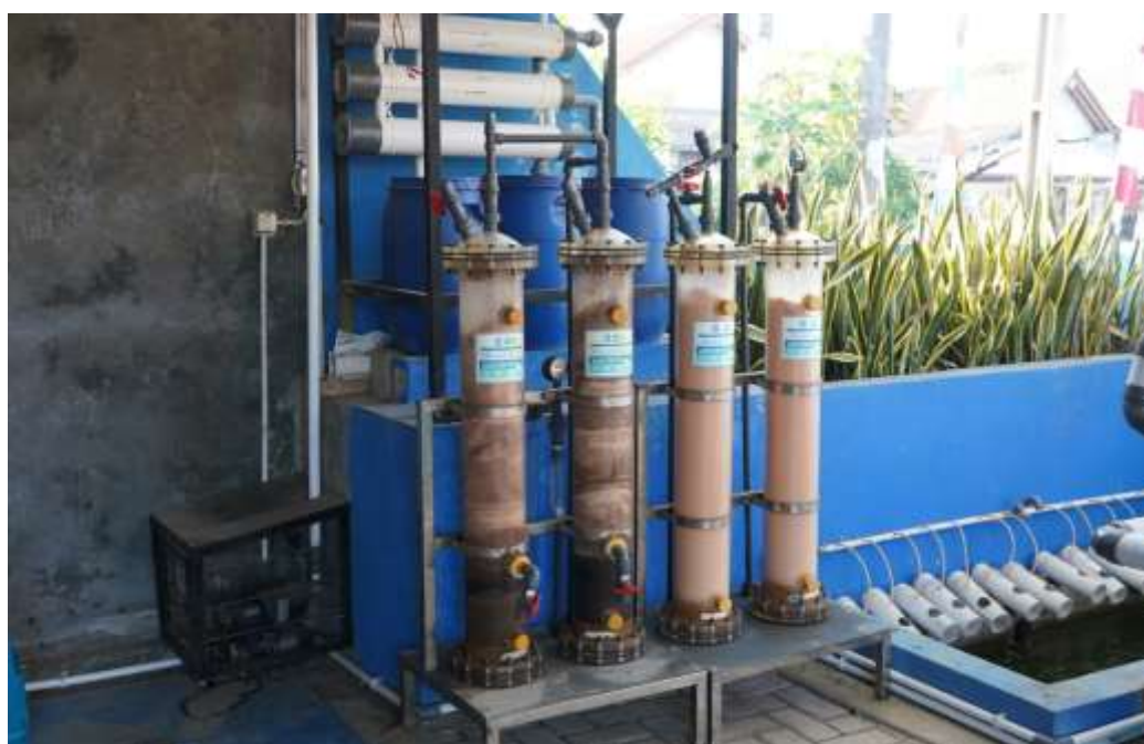
Figure 1. Mechanical, biological, and chemical filter
