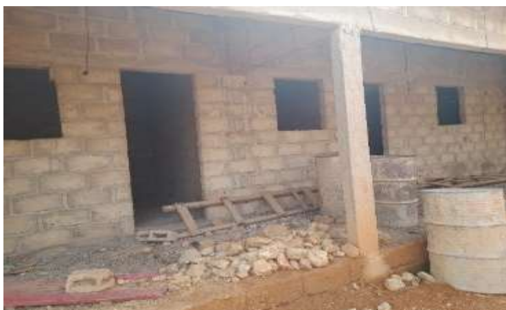
Photo 4 : Modern building under construction in Boyo
