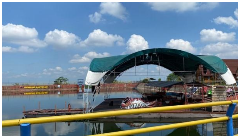
Figure 3. Asih Swargaloka Embankment Facilities Today
